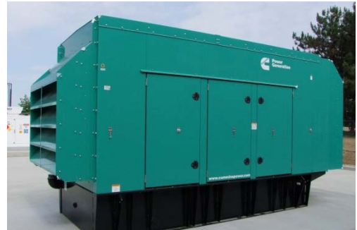
A power generator that can supply electricity to the CNG station in the event of a power outage. Photo from Marathon Technical Services, NREL 30346
