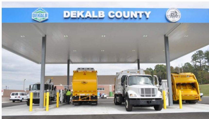
This CNG fueling station in DeKalb County, Georgia, dispenses RNG made from landfill gas. Photo from Robert Gordon, DeKalb County, NREL 26760
