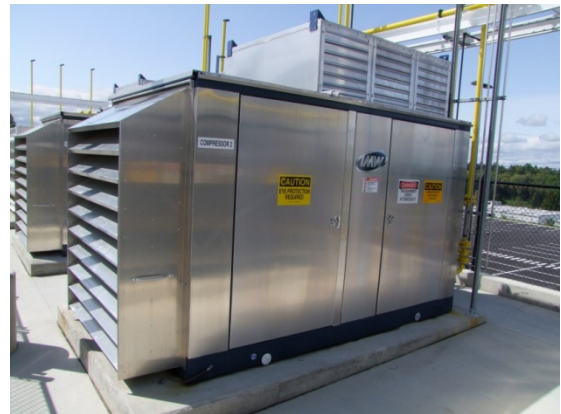
Two enclosed compressors, protected from inclement weather. Photo from Marathon Technical Services, NREL 30343
